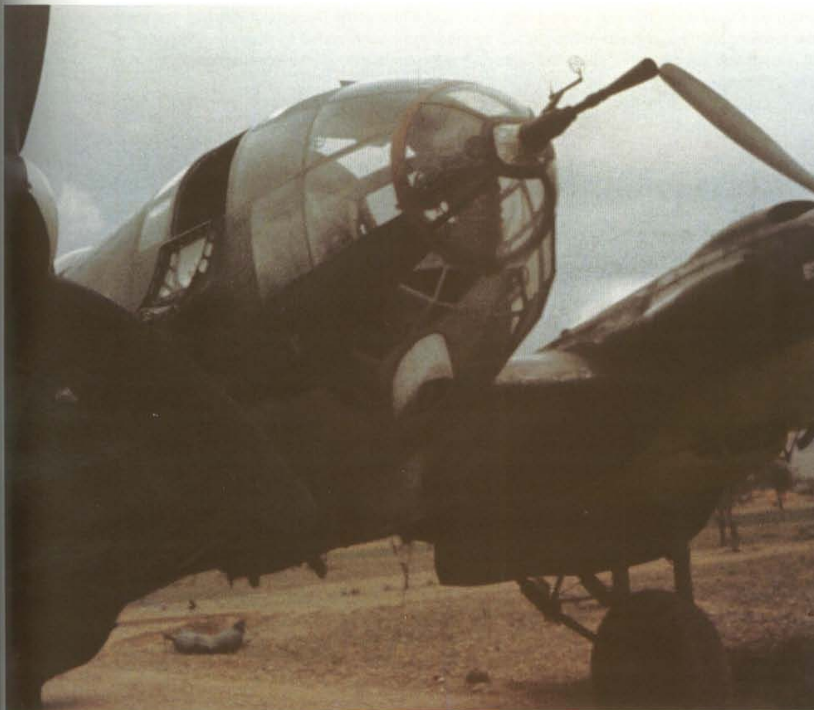
LEFT: This colour photograph of an He 111 H-6 was taken at Kalamaki, Greece in 1943. The aircraft belonged to 5./KG 100. Note the yellow painted lower engine cowls, red painted circular framing on the nose glazing and the flash protector over the muzzle of the MG 151 cannon barrel.
