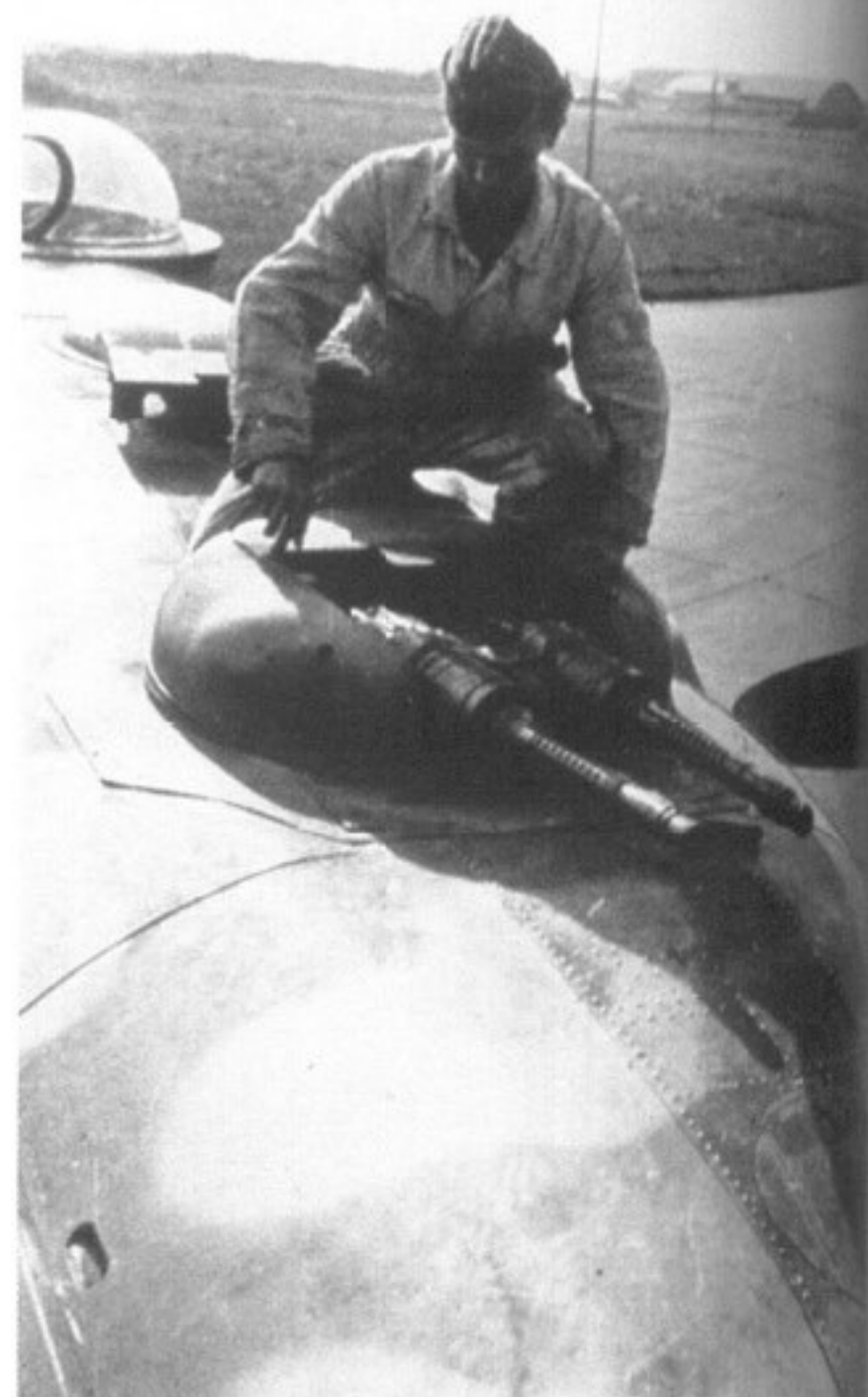
ABOVE: A ground crewman services the twin remotely-controlled MG 131 machine guns in the B1-stand atop a He 177. This turret was controlled by the gunner in the dome-like cupola behind.
